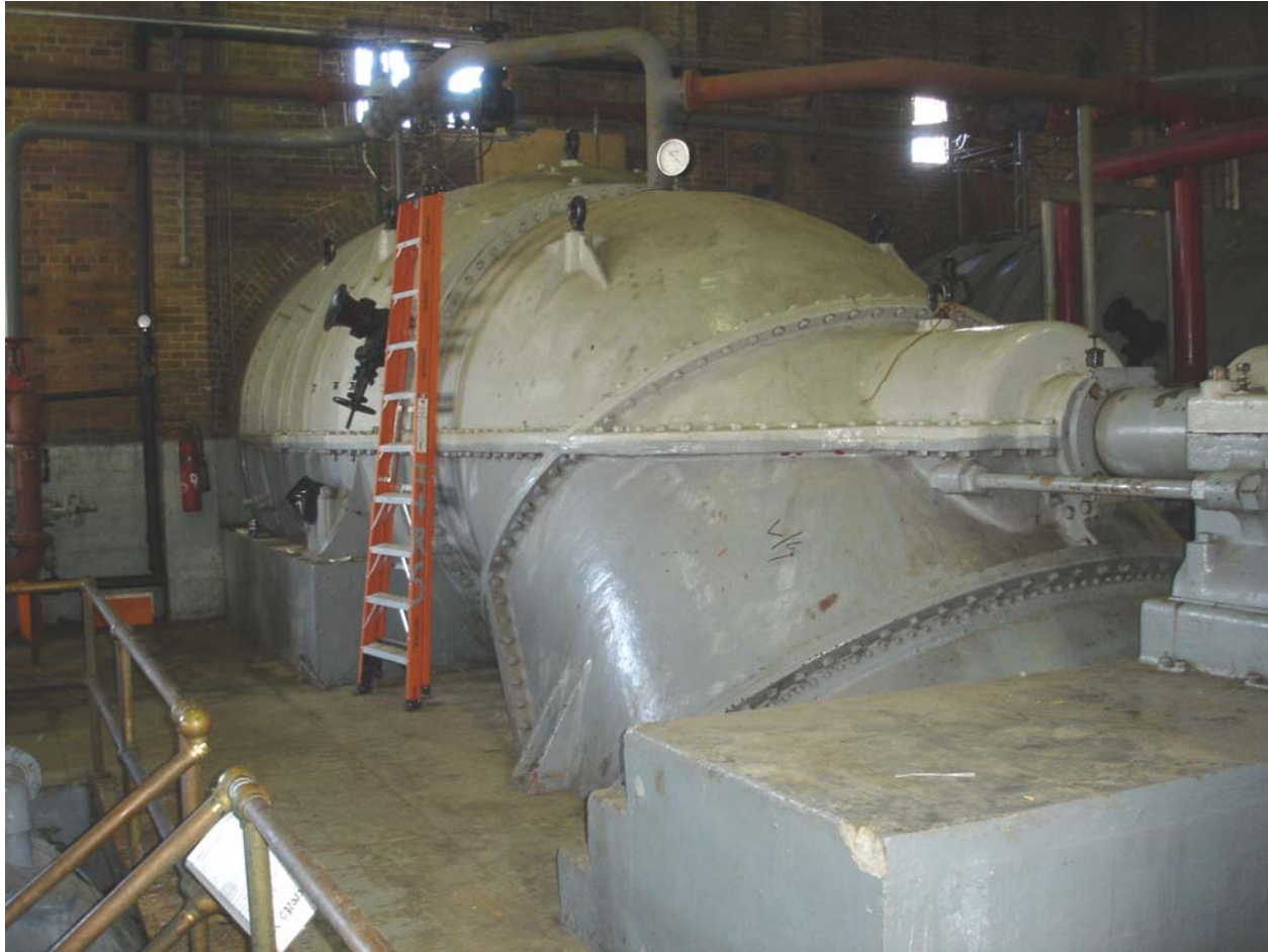
Figure 7. Large Horizontal Shaft Pump
