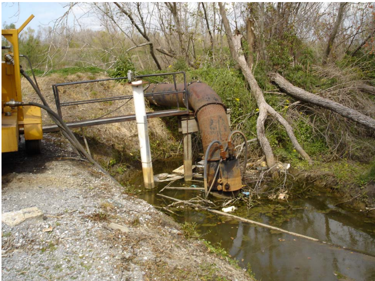
Figure 23. Hydraulically Driven Submersible Pump
